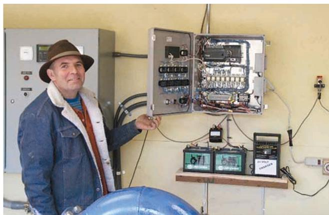
levels. Level options are programmed on a keypad on a secondary control panel, and a digital readout gives water levels in both lakes, as well as a temperature reading of the lakes and Baker Creek.
